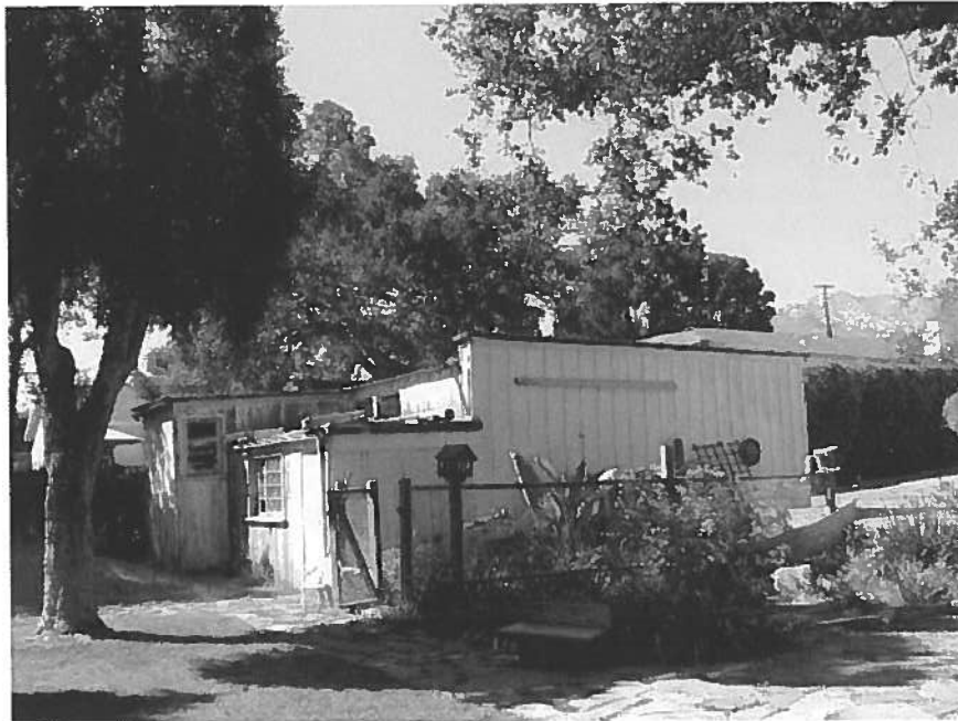
Plate 2. Two-car garage at 2311 Santa Barbara Street, facing northwest Showing rear shed roof wing at left and infill at center Photograph by A. C. Cole, August 1999
