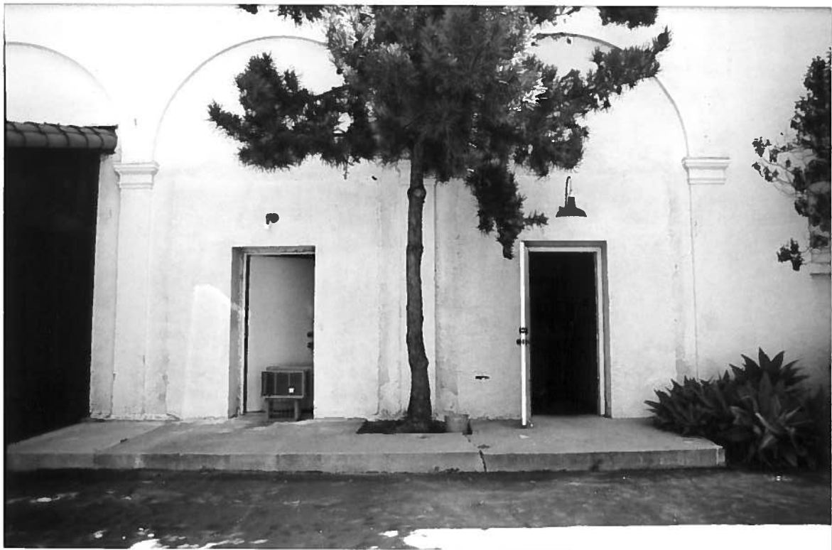
FIGURE 9 West Elevation (Blind arches with inset doors)
